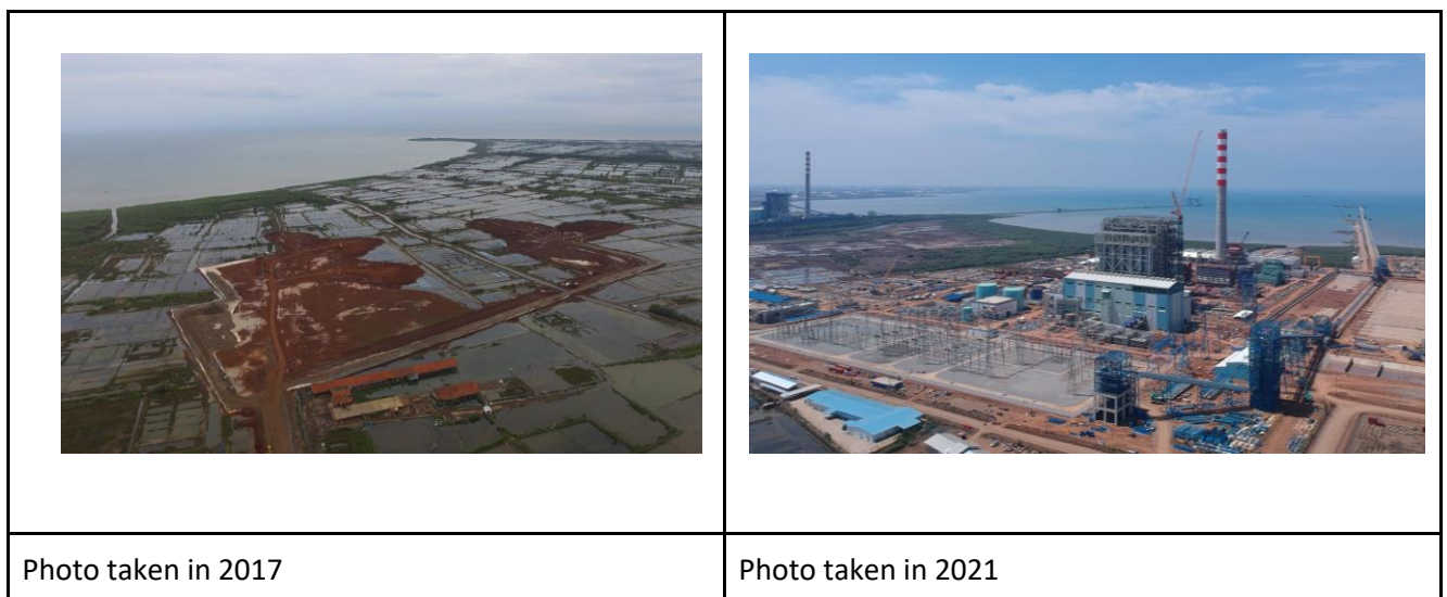
Figure 1. Before and after the construction of PLTU Cirebon Phase 2
